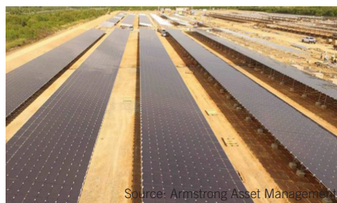
Project 4 & 5 6MW+4MW Site: Installation of Solar PV Modules Na Khok, Samut Sakhon
