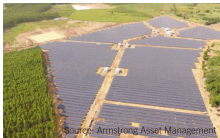
Project 1 & 2: 8MW+8MW Site Installation of Solar PV Modules Srimahapho, Prachinburi
